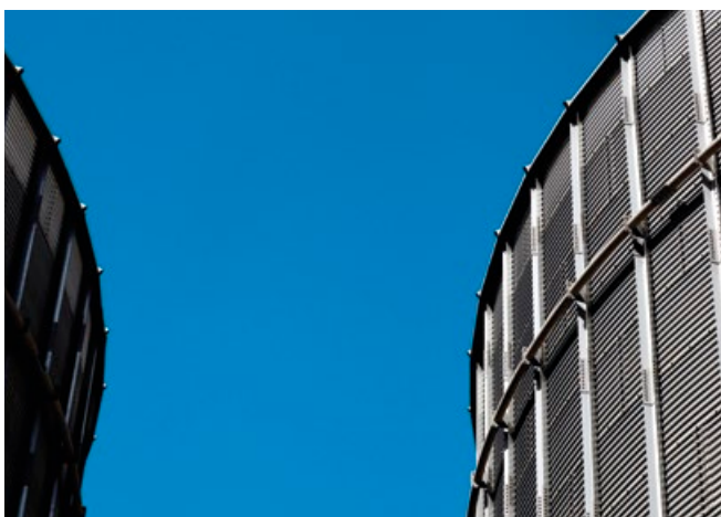
ENG. Detailed view of wind protection rings FRA. Détail anneaux anti-vent ITA. Particolare anelli antivento
